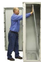
Continue to push top of panel until collar studs protrude through panel mounting holes.
