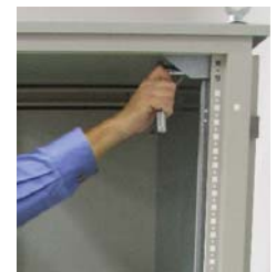
Secure panel to studs.
